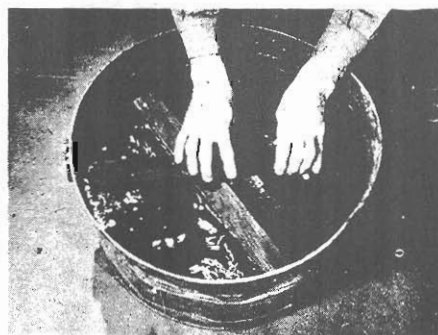
Soften the cross pieces for bending by soaking them in water. It will take about 24 hours in cold water, a few hours only if water is hot.
